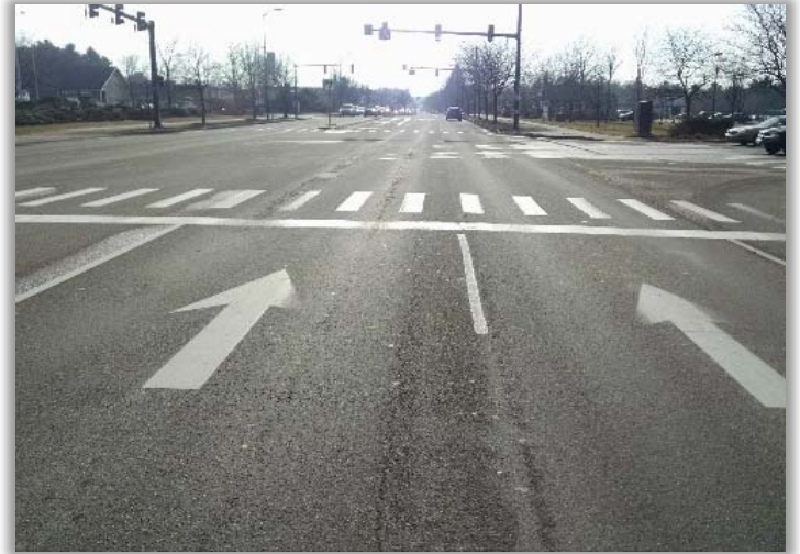
South Burlington – Dorset Street – Pavement Evaluation
