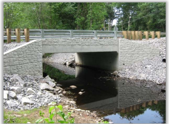
Drew Road Culvert Replacement – Derry, NH
