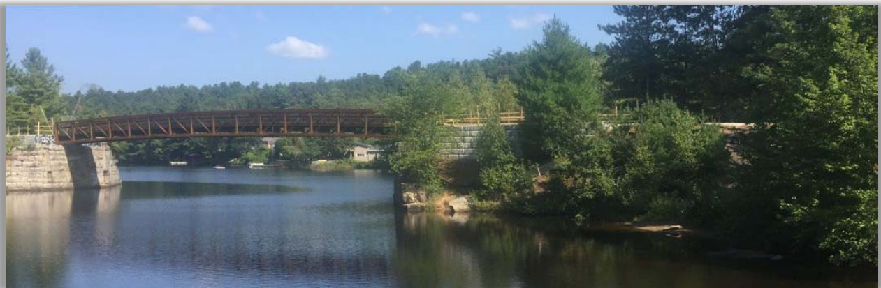
Manchester, NH – Piscataquog River Trail – Pedestrian Bridge
